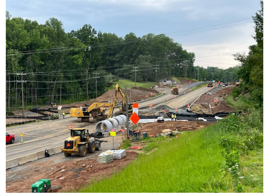
Pipe replacement under Route 29 (June 2025)
